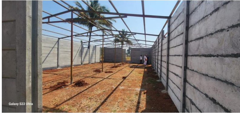
Ghoshala construction in progress
